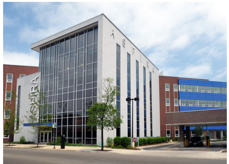
US GBC LEED Gold certified Aspira Business and Finance High School. New 81,000 sf high school construction project.
